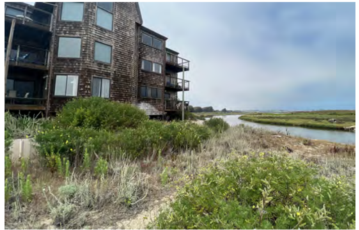
Photo 84: Sheetpile wall southeast of Pelican Drive - Complex E
