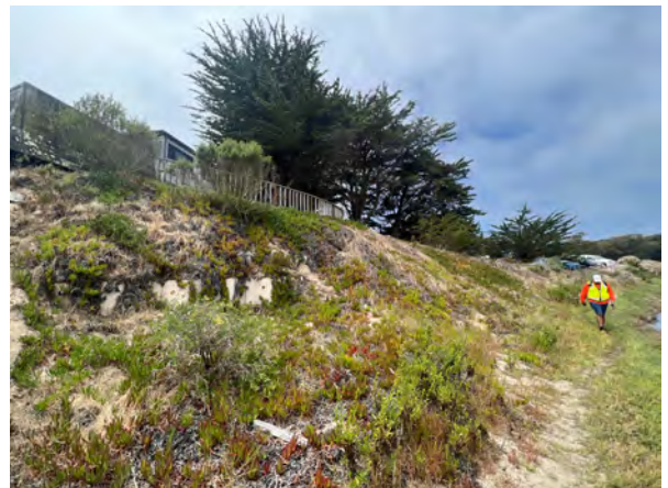
Photo 86 Sheetpile wall northeast of Pelican Drive - Complex E
