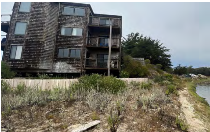
Photo 85: Sheetpile wall east of Pelican Drive - Complex E
