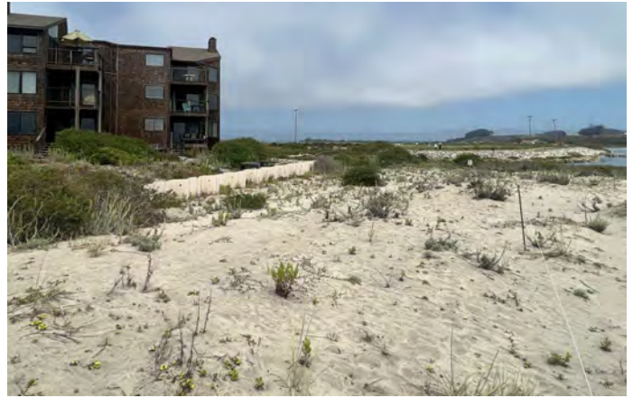
Photo 83 : Sheetpile wall south of Pelican Drive - Complex E
