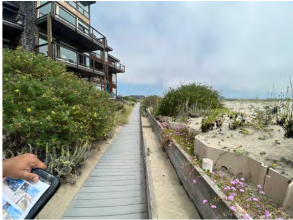
Photo 82: Sheetpile wall south of Pelican Drive - Complex D
